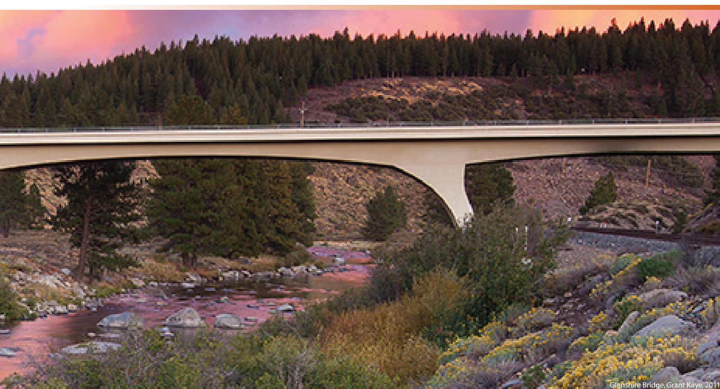
Glenishire Bridge, Grant Kaye, 2011
